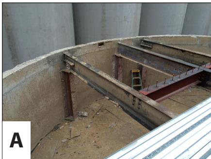
A New support beams (A) replaced some older, out-of-place beams, with some old beam material used to support the new beams. Metal sheeting (B) and 60-grade rebar (C) was installed as the foundation for a new concrete roof deck. New roof deck (D) was treated to resist water and further deterioration. Photos courtesy of C-TEC AG.
